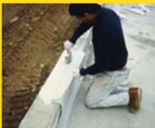
D) 1° application brush and a mixture pose tissue
