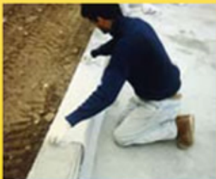
D) 1° application brush and a mixture pose tissue
