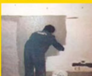
D) 1° application dough and laying fabric wall
