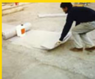
D) 1° application dough and laying fabric wall
