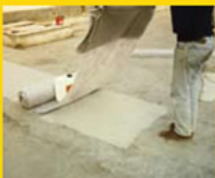
D) 1° application dough and laying fabric wall
