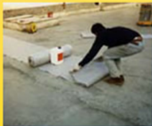
D) 1° application brush and a mixture pose tissue
