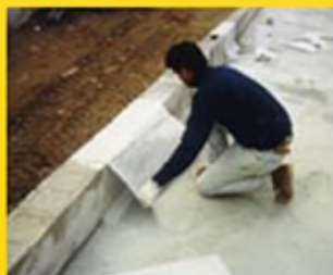
D) 1° application brush and a mixture pose tissue
