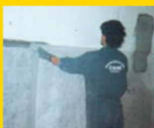
D) 1° application dough and laying fabric wall
